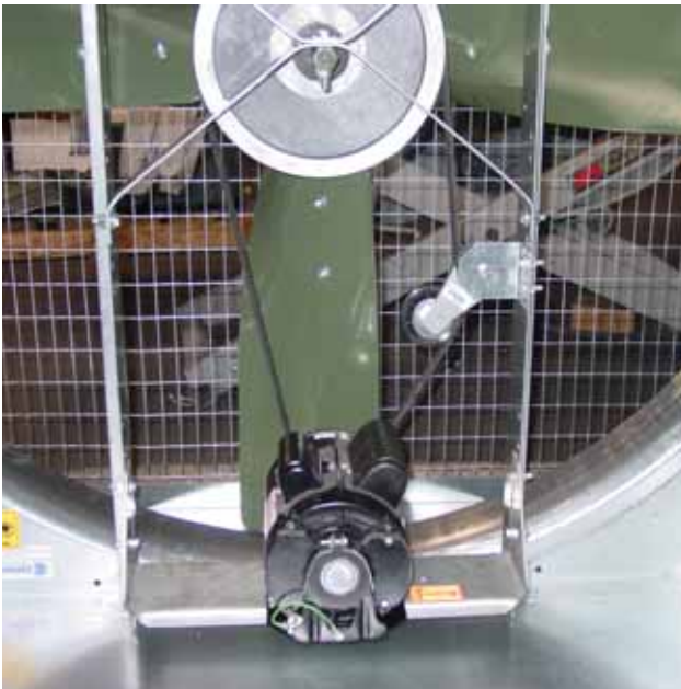
NEFB52 with motor mounted at the bottom of the fan
