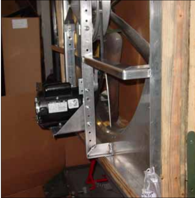
AL48 with motor mounted at the bottom of the fan
