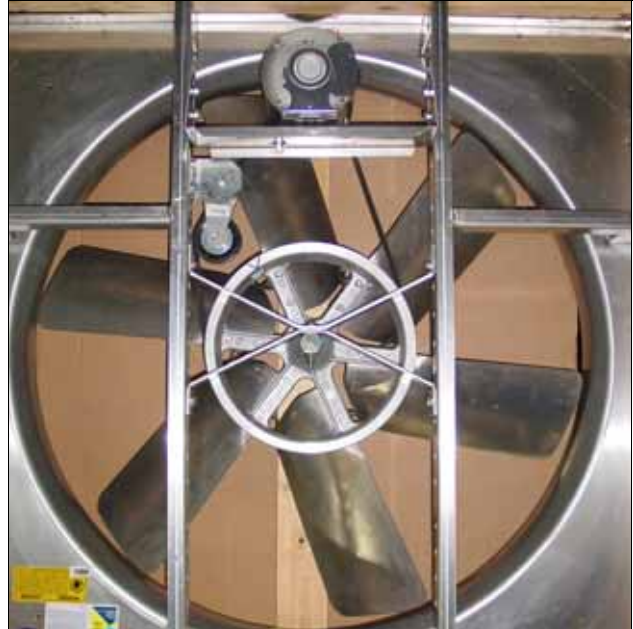
AL36 with motor mounted at the top of the fan
