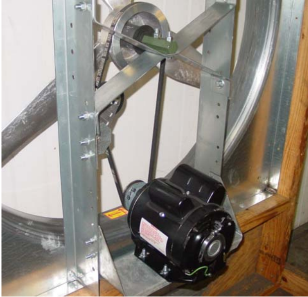
NBC36 with motor mounted at the bottom of the fan
