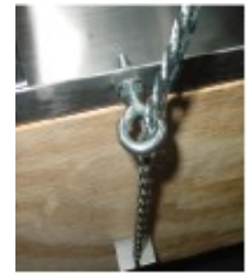
Figure 3 Manual Chain Eyebolt
